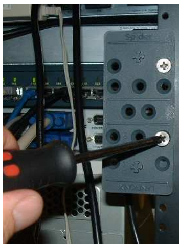
1. Mount the bracket with a Phillips-head screwdriver
