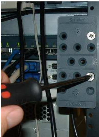
1. Mount the bracket with a Phillips-head screwdriver
